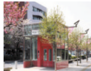
Elevator at Sakura-shinmachi Station
