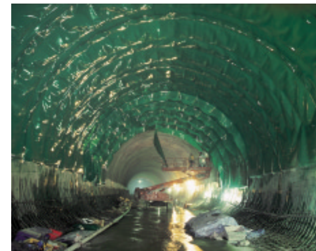
Wrapping the lining of the tunnel in a waterproof sheet
