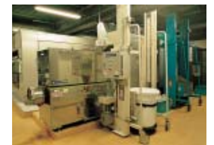
Kitchen waste disposal equipment
