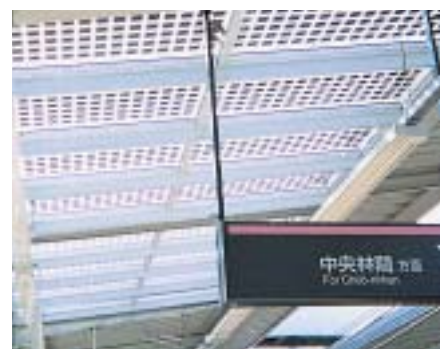
The experimental installation of solar power generation
